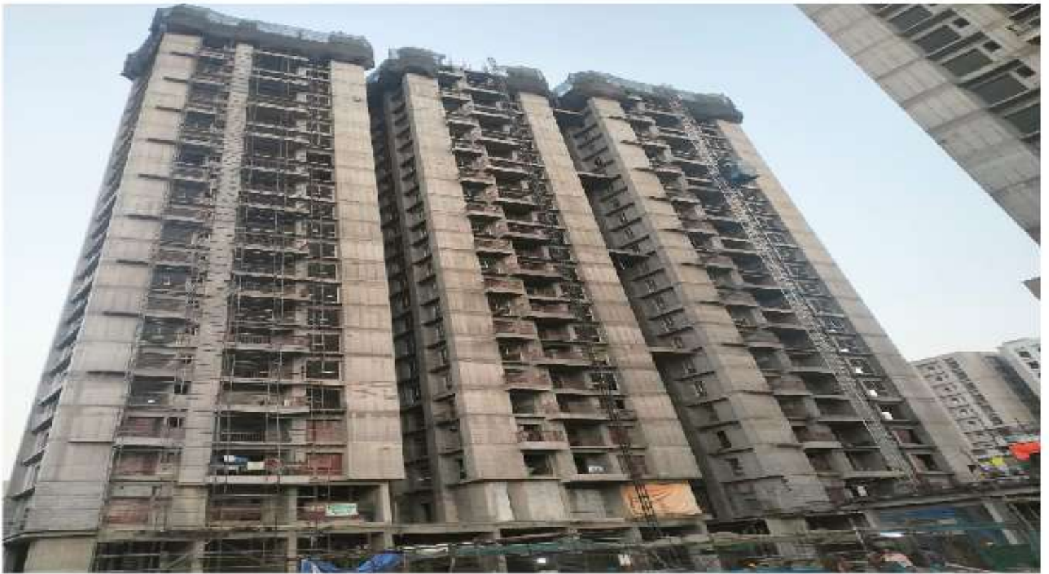
BLOCK 3 :: ABOVE ROOF STRUCTURE IN PROGRESS
